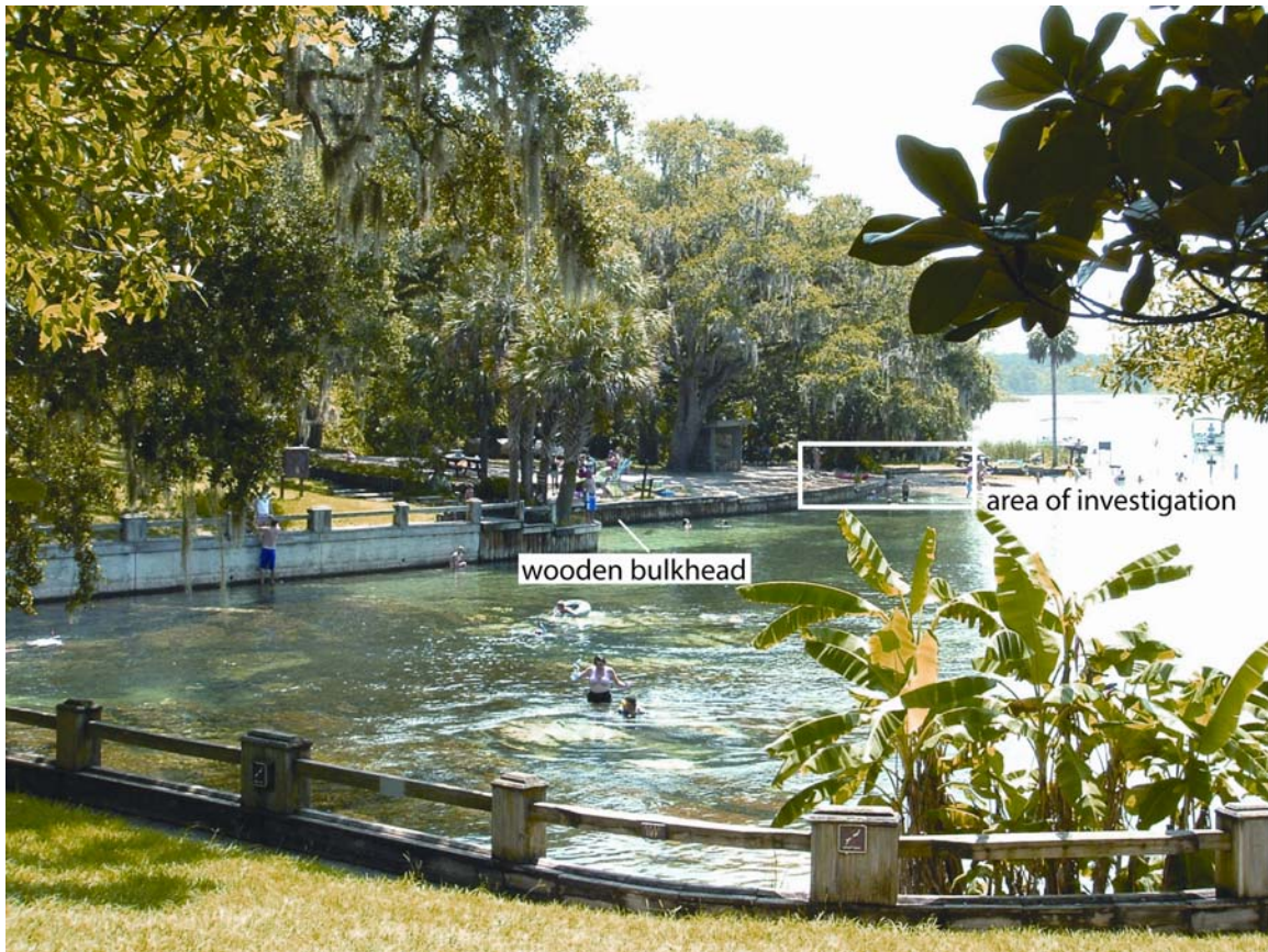
Figure 1-2. View of Salt Springs Recreation Area facing northeast, showing location of wooden bulkhead and area of archaeological investigations by NPS and LSA (ca. 2006 photo modified by author from http://travel.webshots.com/photo/1546028957084561839csjRcT ).
