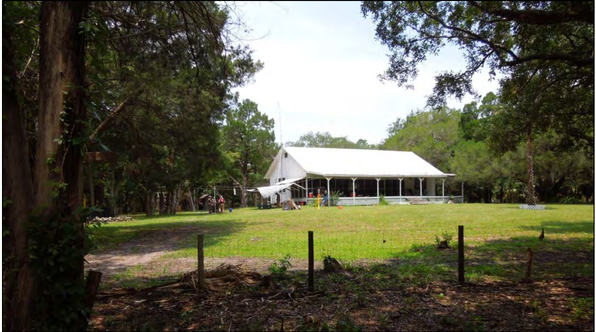
Figure 1-2. Restored cypress log hunting lodge located on Dan May Island.
