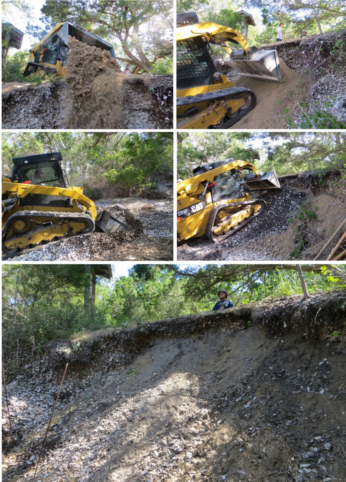
Figure 2-13. Photographs of the process of backfilling the escarpment of the south ridge at Shell Mound (8LV42): dumping aggregate from the top (upper left); pushing aggregate up escarpment (upper right); scraping up displaced shell (middle left); emplacing shell on escarpment (middle right); final scree slope of emplaced fill (bottom).
